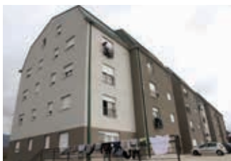
Construction of 62 apartments Niksic, Montenegro
