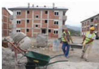
Construction of 120 apartments Konik Camp, Montenegro
