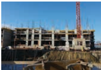
Construction of 235 apartments in Ovca, Belgrade
