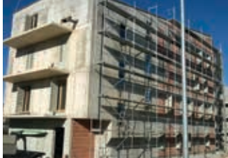
Construction of 40 apartments Knin, Croatia
