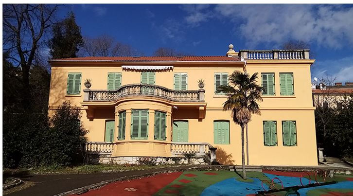
Energy renovation of preschool education subcentre Vidrica
